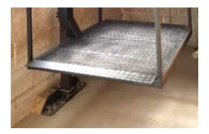
15.5. When attaching a Column to an Armless Base be sure **the seam on the Column faces to the right or left, not to the front or back**. And the vertical flange must face the wall or support it will be bolted to.
