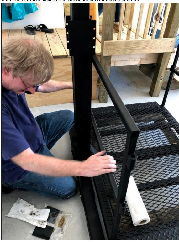
19.9. Ensure that the large slip pad has not fallen out. Insert one of the smaller slip pads into the pockets on each side of the Collar. If they are a bit tight you may need to tap them with a hammer and screwdriver, or jiggle the Platform.
