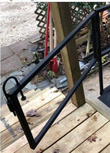
37.5. You can detach easily detach a gate and switch the side it hinges from.
